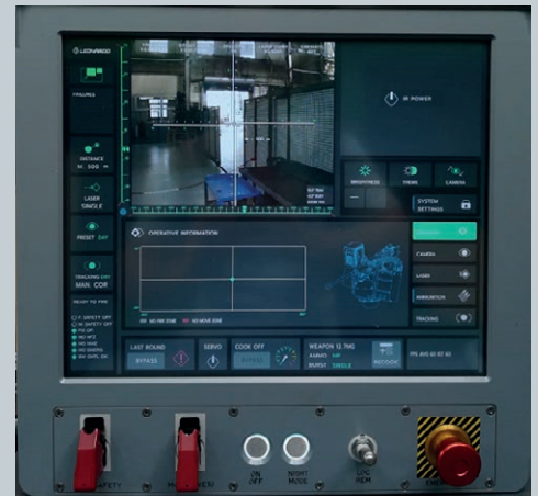
Local Control Panel
